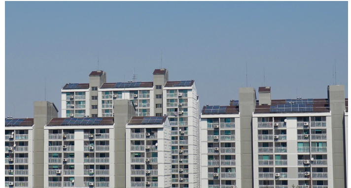
Solar panels installed on existing buildings in Cheongju (Shutterstock)
